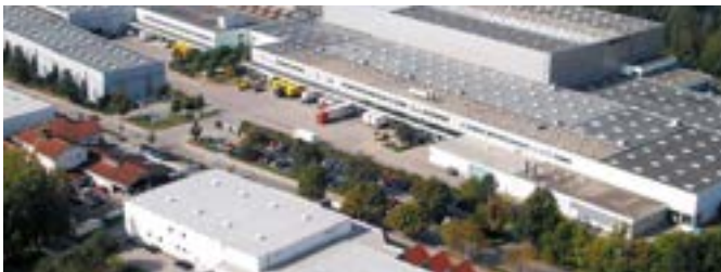
Häfele Distribution Centre Nagold, Germany
