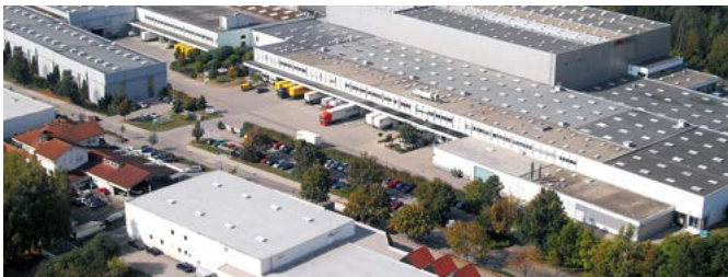
Häfele Distribution Centre Nagold, Germany
