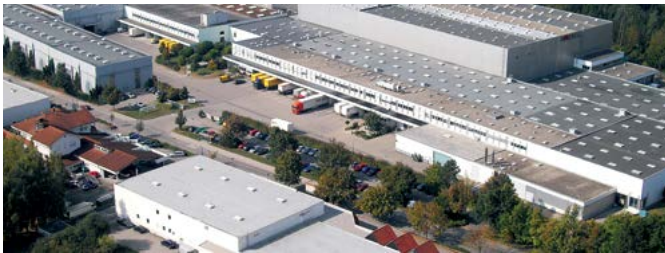
Häfele Distribution Centre Nagold, Germany
