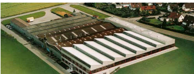
Häfele Production Plant Jettingen, Germany
